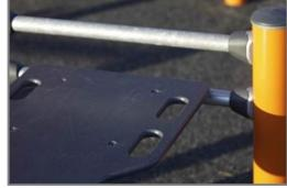
The surface is made of Ekogrip<sup>™</sup> panels, consisting of 15mm polyethylene with a 3mm top-layer of thermoplastic rubber. The Ekogrip<sup>™</sup> panels have a non-skid effect for comfortable and safe training at all weather circumstances.
