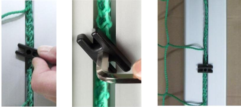
Pull the cord through each net meshes and fix it on both net hoops, if necessary lead it through the bore in the net hoop.
